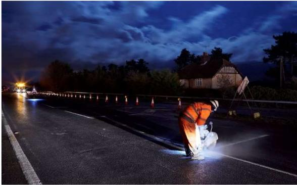
Drying expansion joints before sealing
